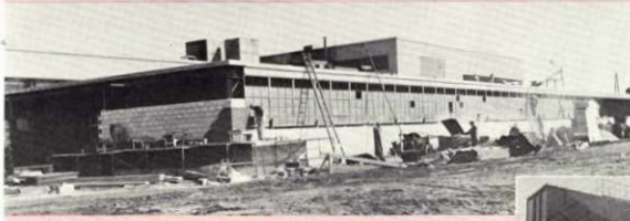
As the new building appeared on April 1.
